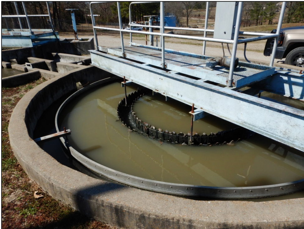
Photograph 6. Secondary clarifier No. 2.
