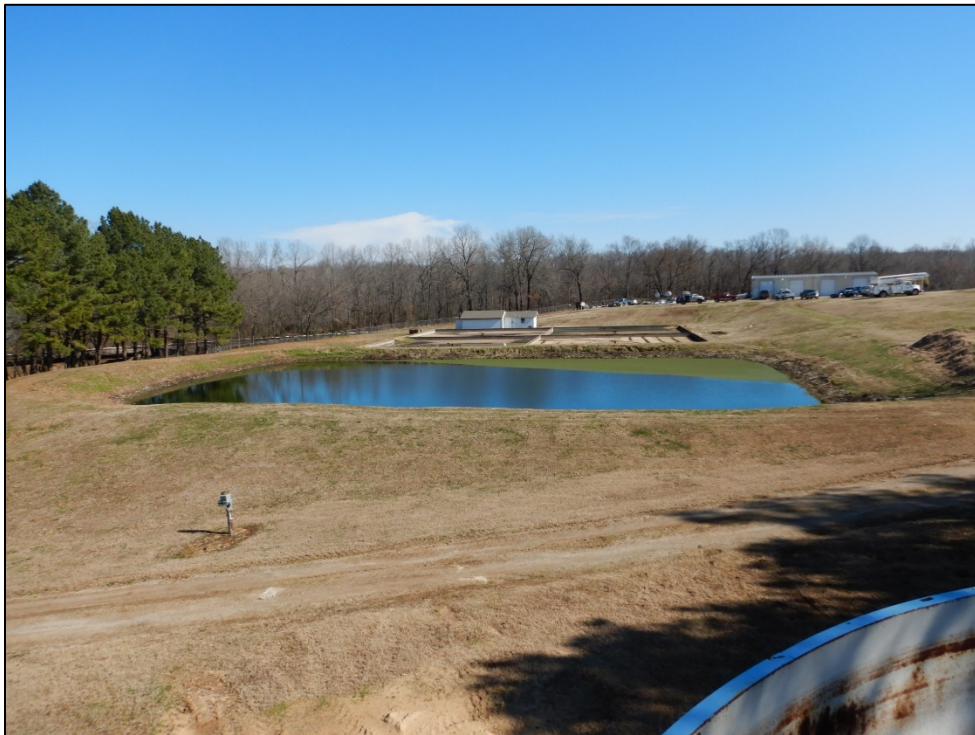
Photograph 2. Equalization basin.
