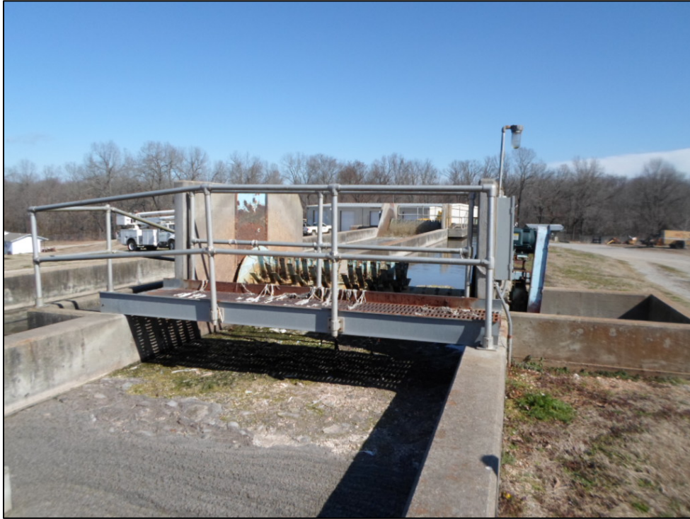
Photograph 3. Oxidation ditch and first rotor. The rotor was not in operation at the time of the site visit.
